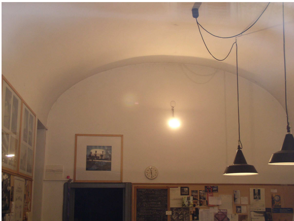
Locale a piano terra
